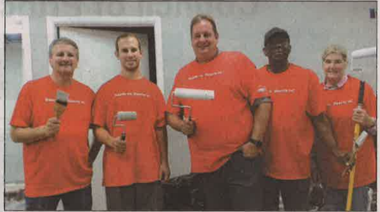
Some of the Lowe's Warrington employees who painted the Opportunity Council building are, from left, Kerry Savrin, Joe Stanton, Aaron Drellich (store manager), Wayne Haynes and Linda Pfeifer.
